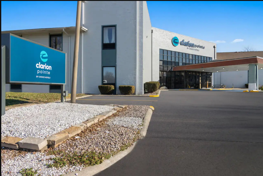
EXTERIOR - PORTE-COCHERE AND BRAND SIGNAGE
